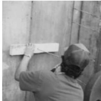
2. A 2x4 wood nailer is included. Fasten it along with the threaded rod directly to the concrete form. This provides support and helps center the complete Cell-Cast® disk assembly.
