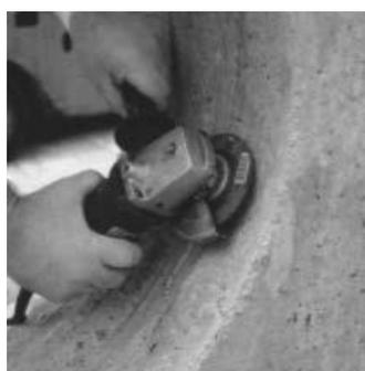
11. Inspect the installation. A smooth opening is important for a proper Link-Seal® modular seal installation. Repair voids and grind smooth any ridges.
