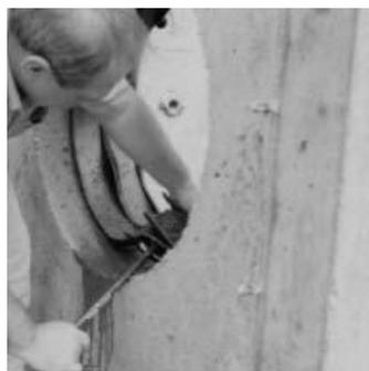
10. Remove disks by breaking out the entire assembly.
