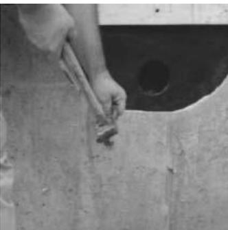
9. Chip excess concrete from the edge of the Cell-Cast® disk assembly and wall.
